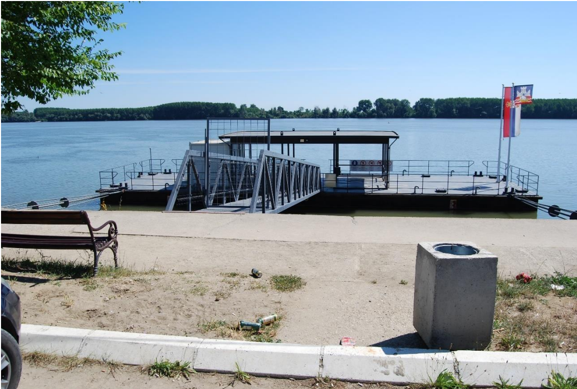
Fig. 48. Pontoon – the dock installed in 2020 Source: archives of the Institute for the Protection of Cultural Monuments of Serbia
